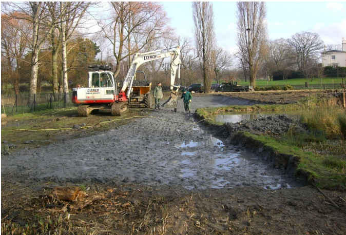
Construction starts on the extension
